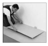
Place a row of full-size 4 mm panels (clear adhesive downwards) overlapping the second row of the 3 mm panels halfway. Install the remaining panels, covering the whole area in this manner.
