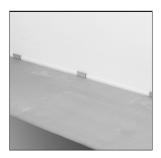
Place a row of full-size 3 mm panels (coloured adhesive uppermost) staggered against the first row of the cut the panels - ideally in a brick design as shown above.
