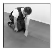
Cut the Forbo foam to fit the floor area and place it on the floor aluminium side upwards. Join the seams with the overlapping aluminium tape.
