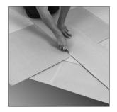
Forbo QuickFit can be cut from the top using a straight cutting blade, and then snapped.
