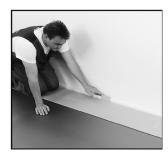
Maintain a gap of at least 6 mm between panels and walls. Start at the shorter wall of the room with a row of 3 mm panels cut in half lengthways (coloured adhesive uppermost).
